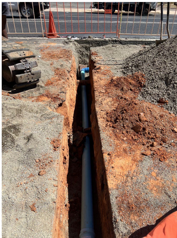
Figure 2: A new fire hydrant was installed in Narromine for Fire and Rescue
