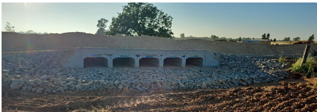
Figure 5: Recently completed culvert on Lincoln Lane
