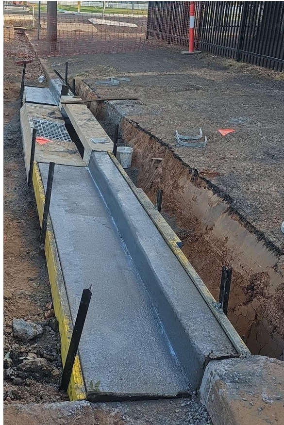
Figure 11: New stormwater inlet has been installed in front of the school
