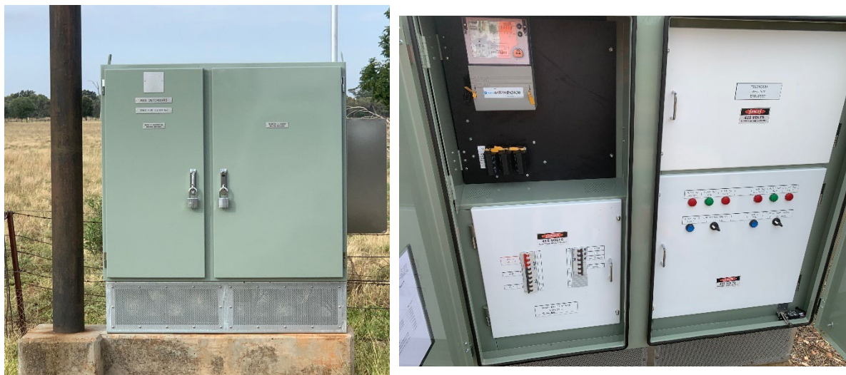
Figure 1: New electrical switchboards installed at Trangie's four sewer pump stations, with SPS 3 pictured. Left: External view; Right: Internal view.
